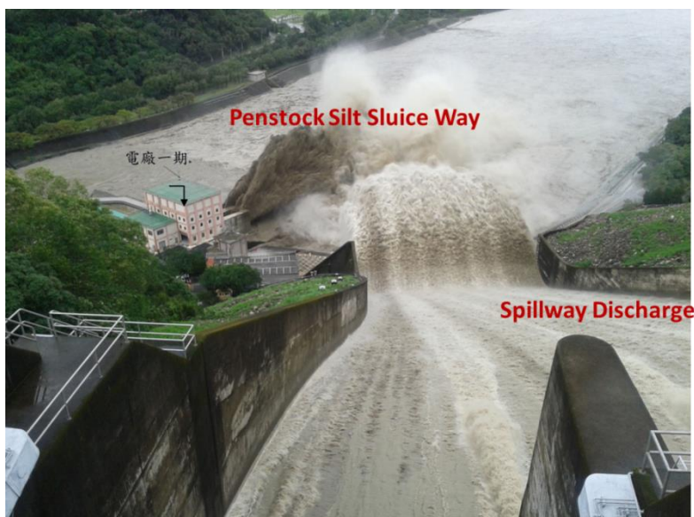
Photo 2 Operation of Spillway & Penstock Silt Sluice Way During Typhoon Soule
