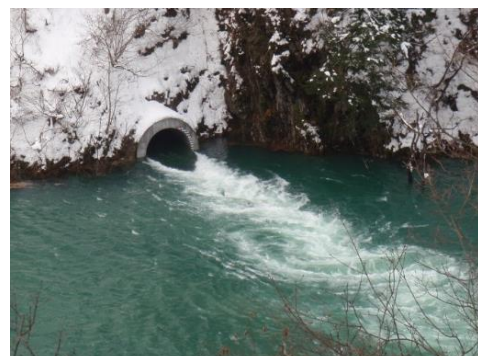
Fig.10 The outlet of tailrace tunnel
