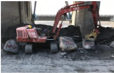
Large rocks at upstream of the weir
